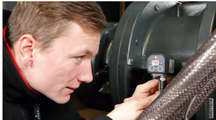
Figure 3 Commissioning of FAG SmartCheck
